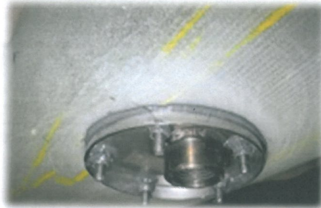
Lower flange of the fuselage fuel tank sealed with ProSeal
